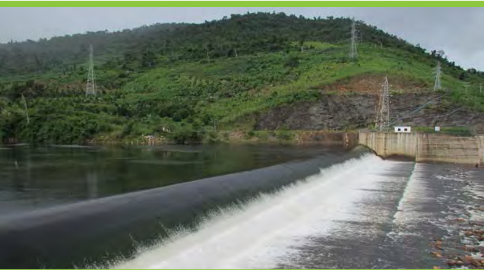
Lower weir, 193 MW Kamchay Hydropower Plant, Cambodia
