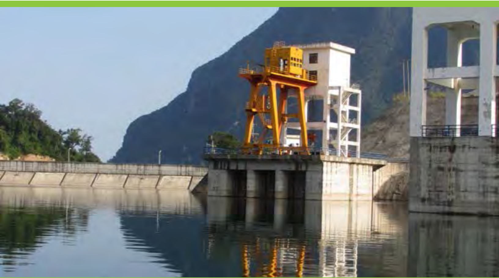
Dam wall with water intake tower of the 100 MW Nam Lik 1-2 Hydropower Plant, Lao People's Democratic Republic
